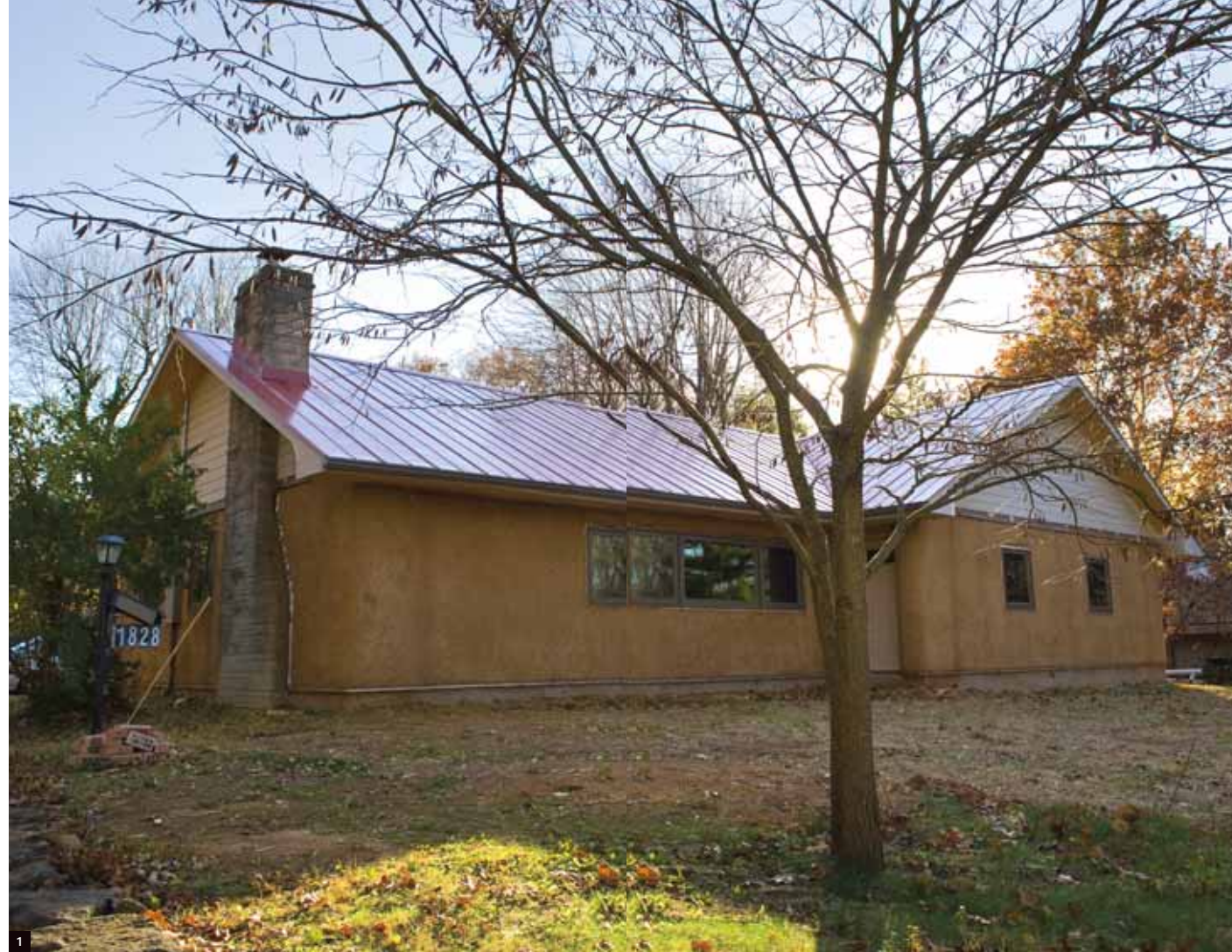
1. The straw-bale "wrap" of this 1940s house has substantially increased its insulation. When finished, the appearance will resemble adobe. A steel roof is ideal for collecting rainwater and can be recycled at the end of its useful life.
