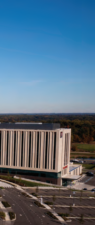
(above) The new IU Health Bloomington at the Indiana University Academic Health Center opened in December 2021; (opposite page, bottom) immediate access to care is now available in Bloomington and Ellettsville at five IU Health Primary Care locations, two IU Health Urgent Care locations, and IU Health Bloomington Orthopedics and Sports Medicine; (below) Dr. Bryan Wohlfeld uses a state-of-the-art augmented reality (AR) tool to perform very precise and minimally invasive spine surgery. Courtesy photos.
